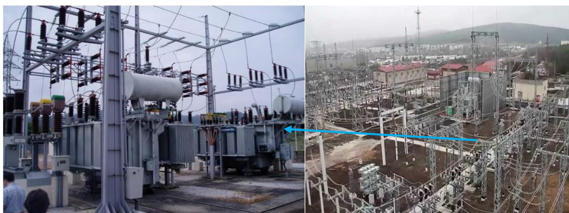
Plate 3.10.1: A Typical AIS Substation (with transformers zoomed in)
